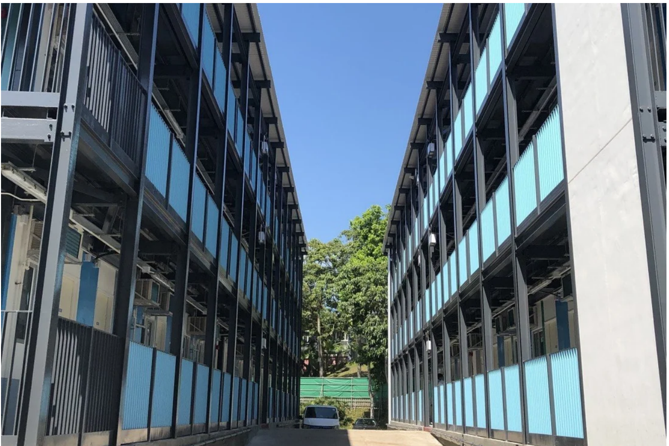
Two of three blocks at a quarantine facility in Sai Kung, Hong Kong, built in 77 days using modular integrated construction (MiC). Several pilot projects are under way in the city, a late adopter of factory built homes. Photo: LWK + Partners
