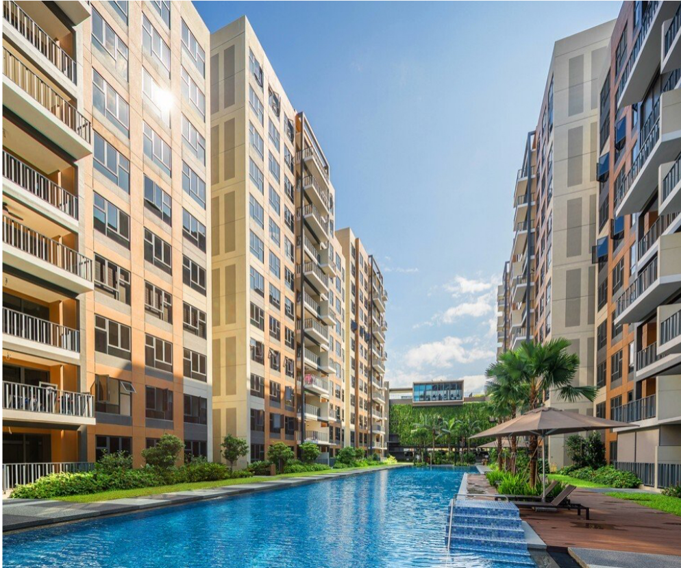
The Brownstone condominium development in Singapore was the first there to be built from precast concrete modules. Photo: Rendy Aryanto/VVS.sg
